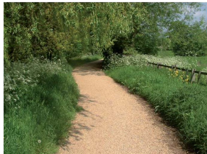
Photo of surface dressed footpath/cyclepath at New Hall Valley Country Park. This type of surfacing is proposed for the majority of the new route.
